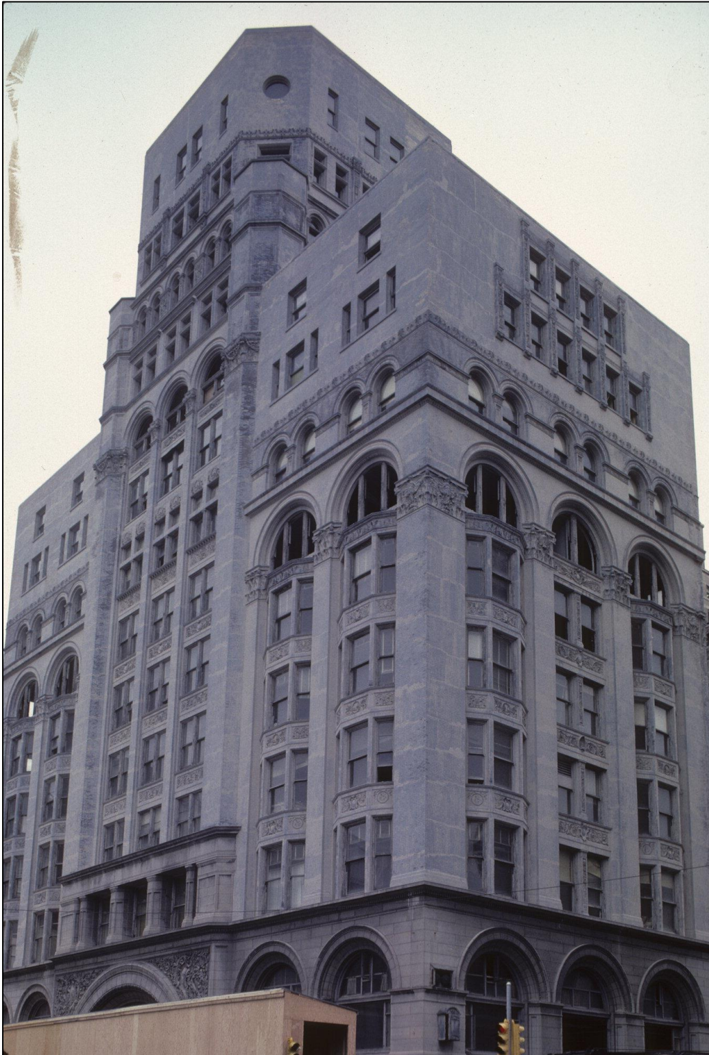
Figure 9. The Pabst Building shortly before demolition. Photo provided by Tim Askin, City of Milwaukee.
