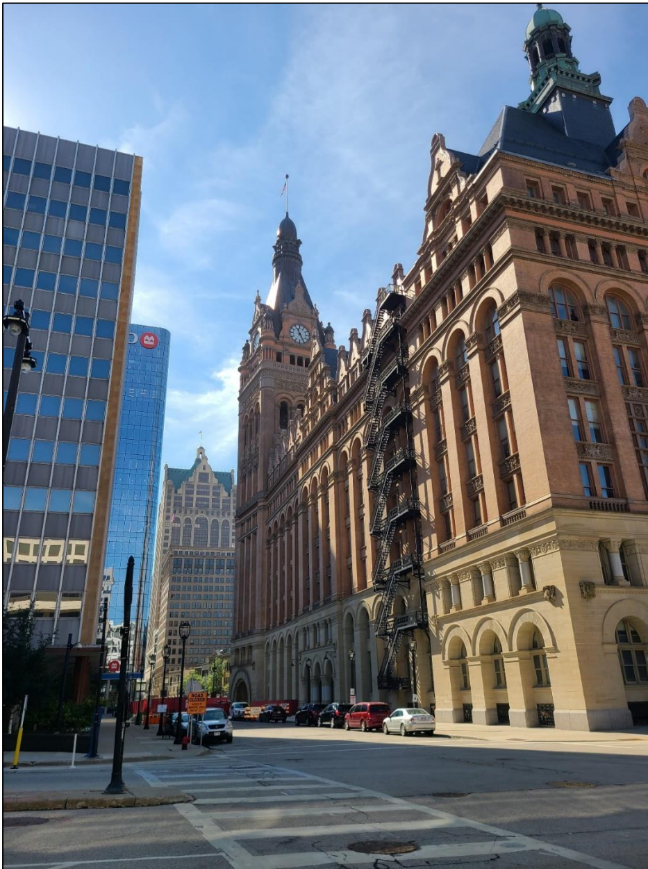
Figure 8. Looking south down North Market Street from Kilbourn Avenue and showing 100 East in context with the historic City Hall in foreground. Photo by Loughlin, October 2022.
