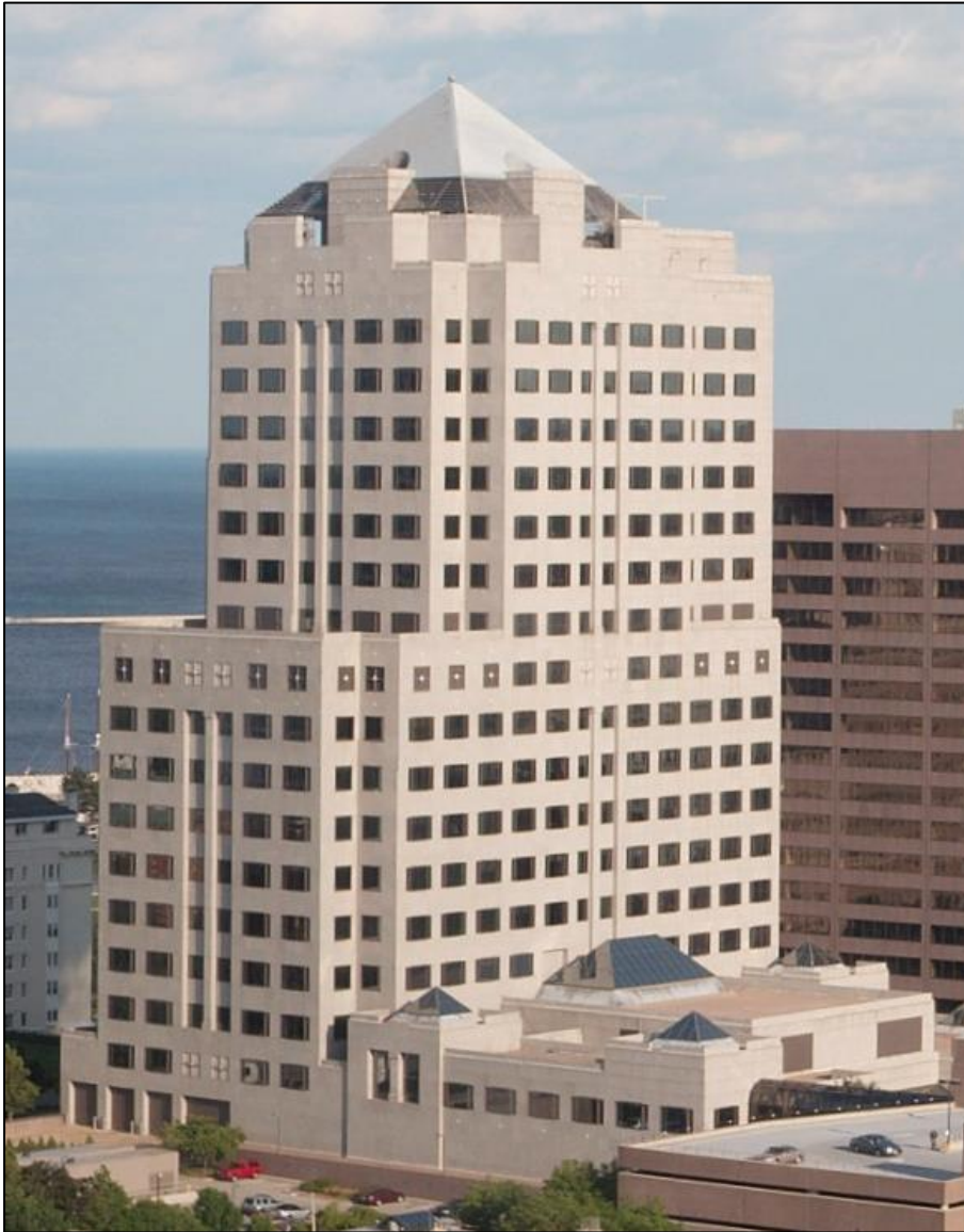
Figure 15. Northwestern Mutual Life Data Center, 818 E. Mason, 1990. Photo from Wikipedia.
