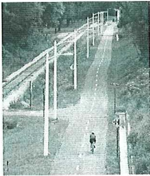
• Figure 26 No barrier between trails users and an active rail line on the Blackhawk Trail in Madison, WI. Photo Credit: Arthur Ross
