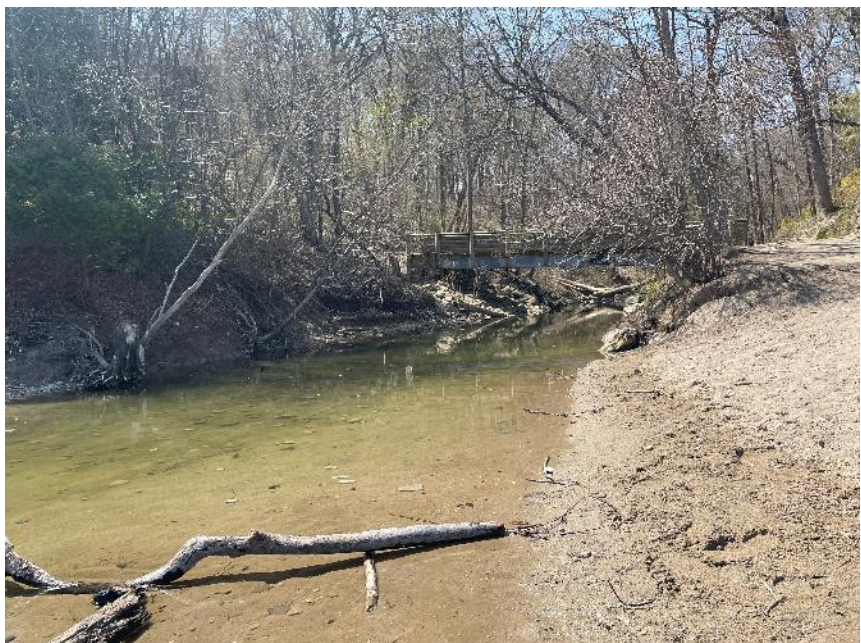
FIGURE 13: A stagnant stormwater drainageway within Grant Park.
