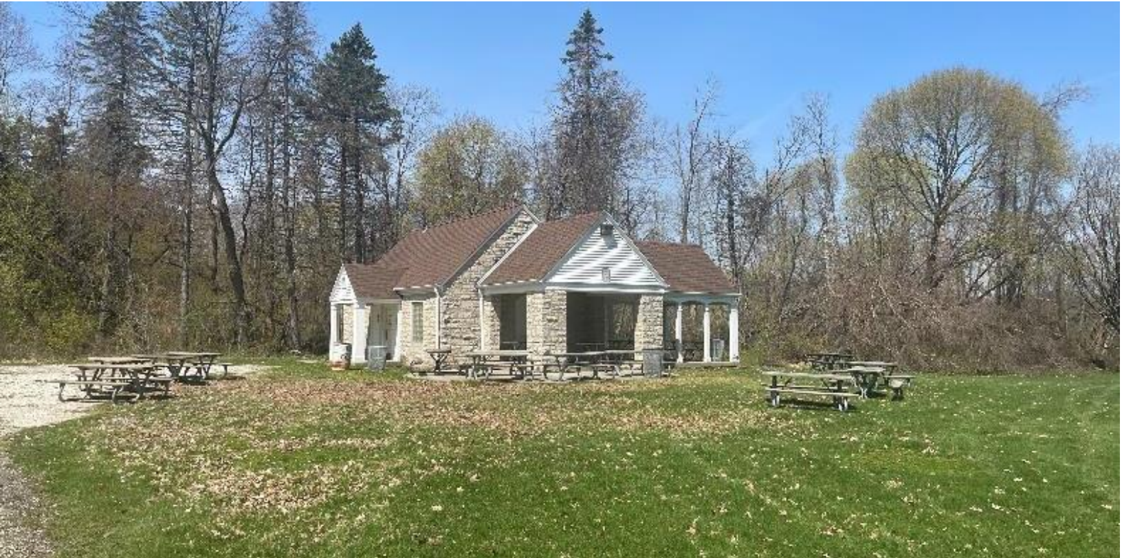
FIGURE 27: If temperatures are warmer, more demand for restroom facilities is anticipated.
