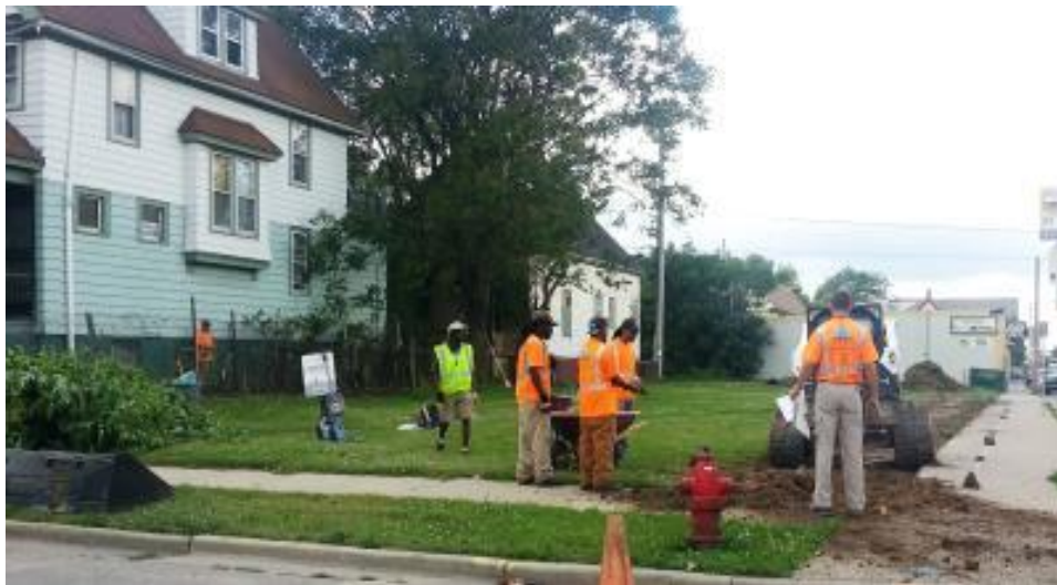
Workers installing green infrastructure
