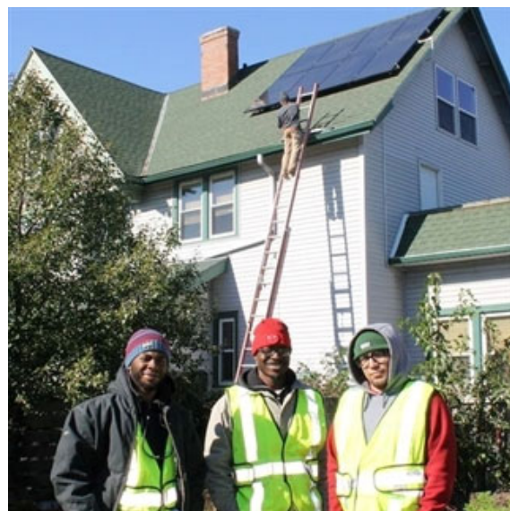
Rooftop solar installation
