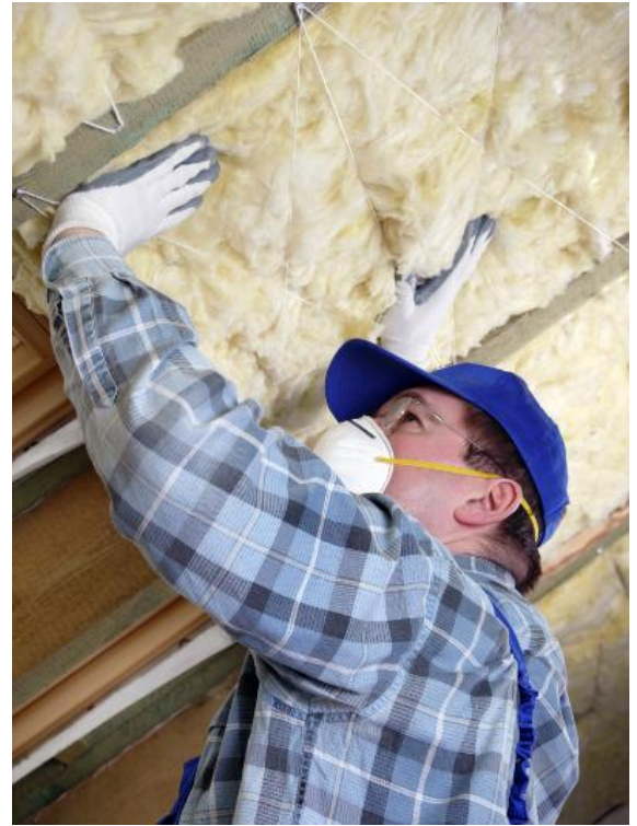
Installation being installed in a home
