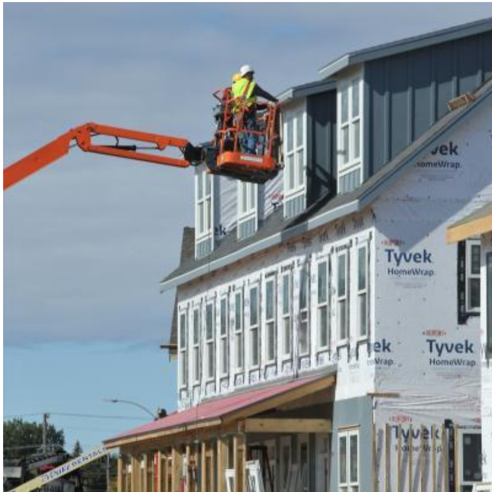
Westlawn Garden modular housing construction
