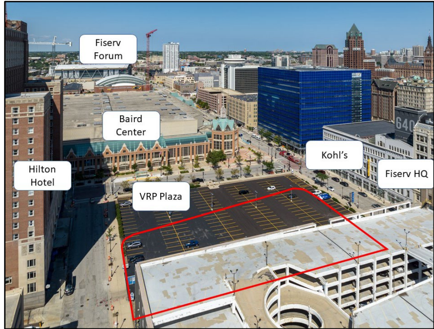
Aerial view of the site
