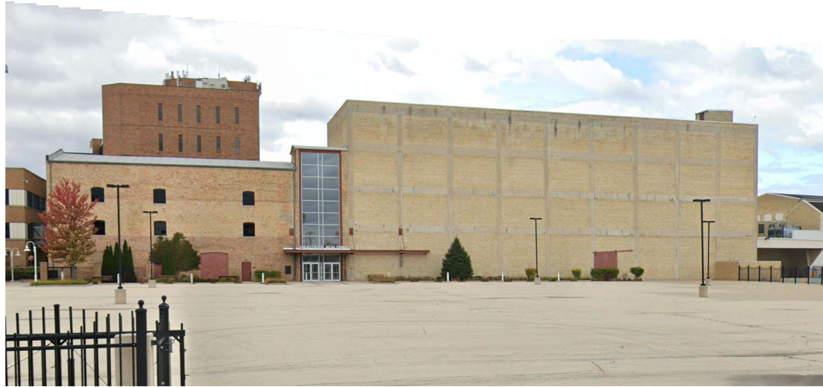
BEFORE- East Elevation of Heritage Building
