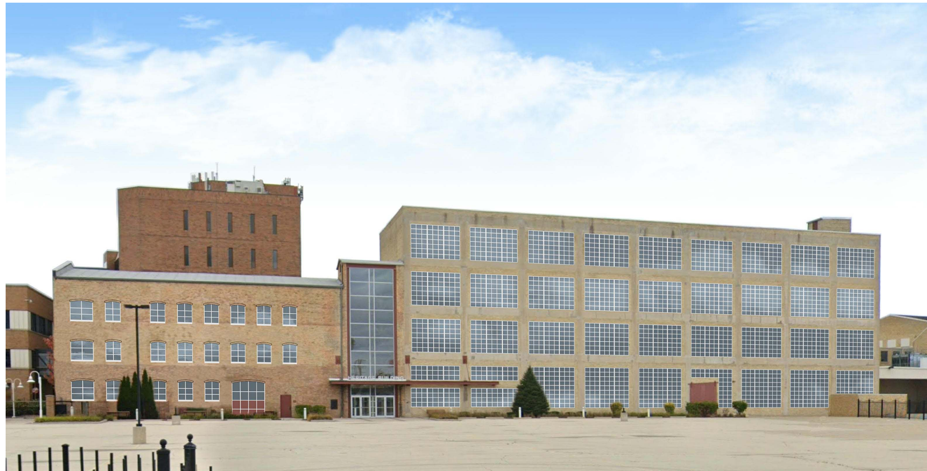
AFTER- East Elevation of Heritage Building
