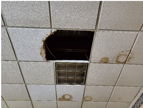
Photo 23: Water damaged ceiling on first floor.
