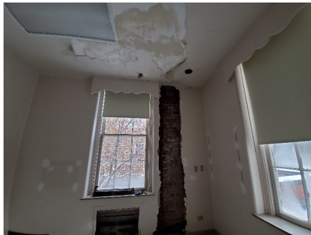
Photo 19: Deteriorated wall and ceiling in Northwest Quadrant.
