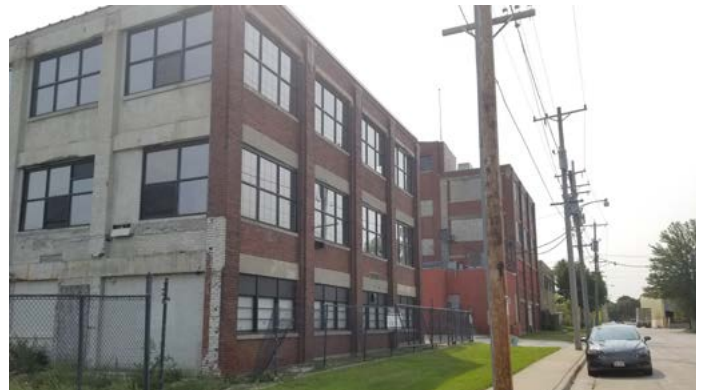
VACANT BUILDING IN RIVERWORKS BID
