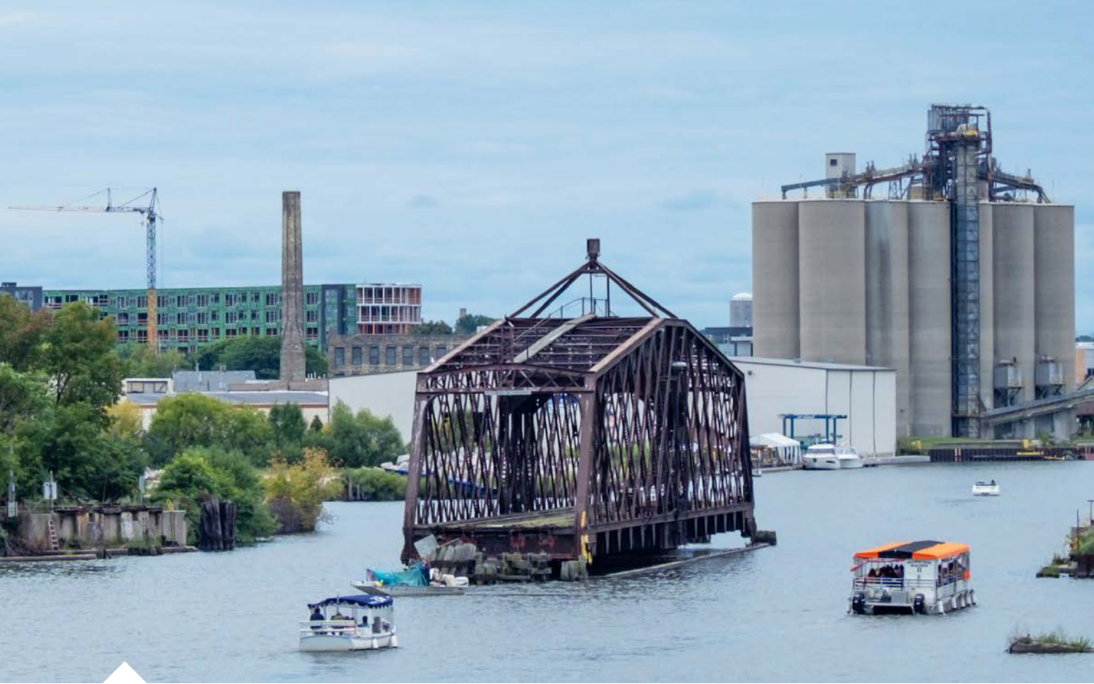
Railroad Bridge , photo by Jiajing Chen
