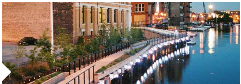
Riverwalk At Metal Sheet Pile River Edge, Historic Third Ward Riverwalk, Milwaukee
