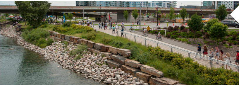
Mixed Type Naturalized River Edge, Riverwalk East Village At Downtown Calgary, Alberta, Canada.
