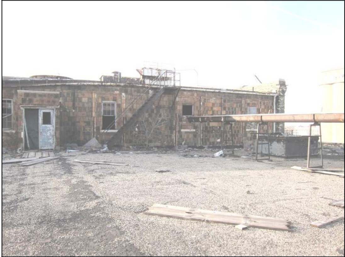
Photo 44: Building 25 seventh floor west penthouse looking west.
