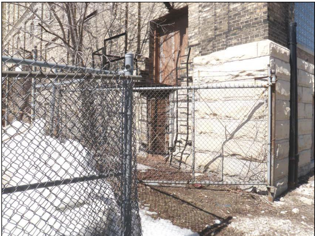
Photo 37: Ground floor of southeast corner of Building 25.
