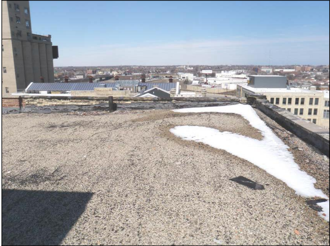
Photo 42: Building 25 roof on seventh floor west penthouse looking north.
