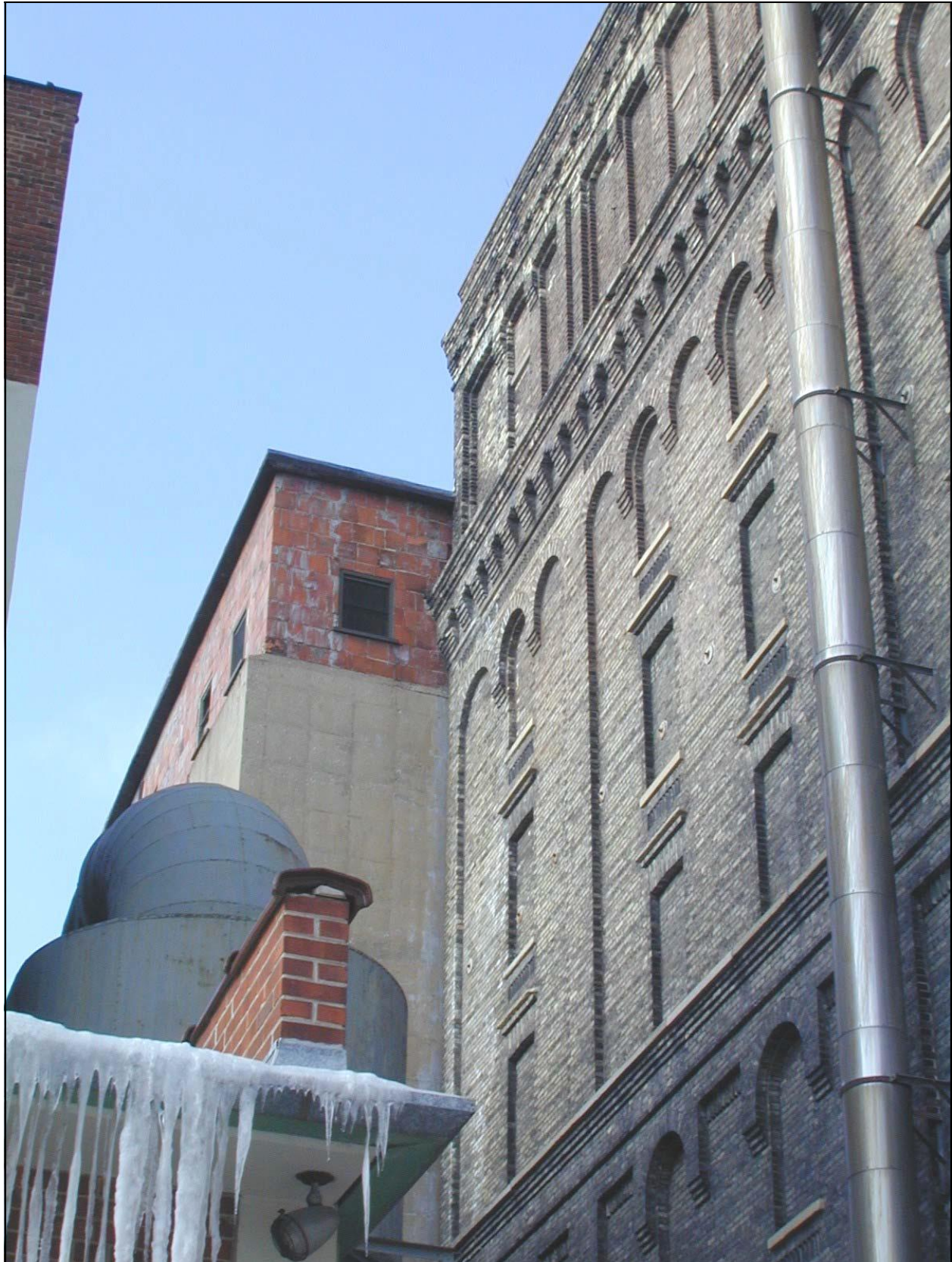
Photo 30: South elevation of Building 24 (left) and Building 25 (right) looking northwest.
