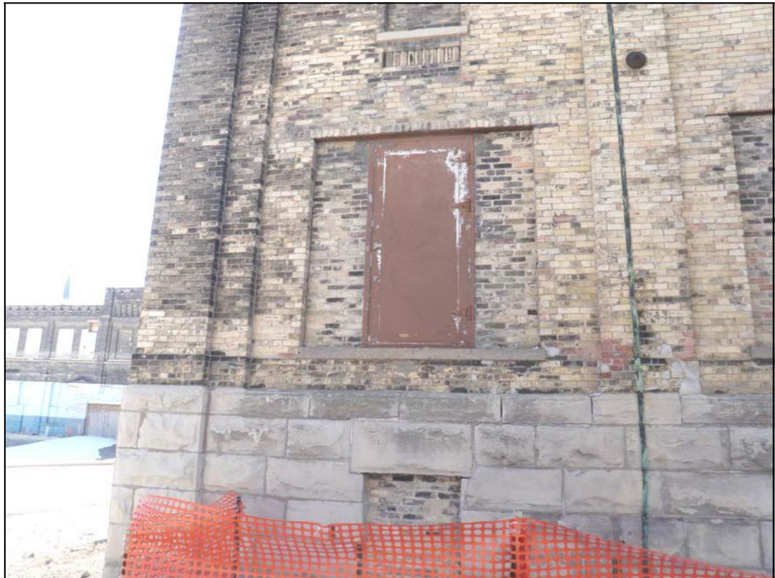
Photo 13: Lower floors of north elevation of Building 25.
