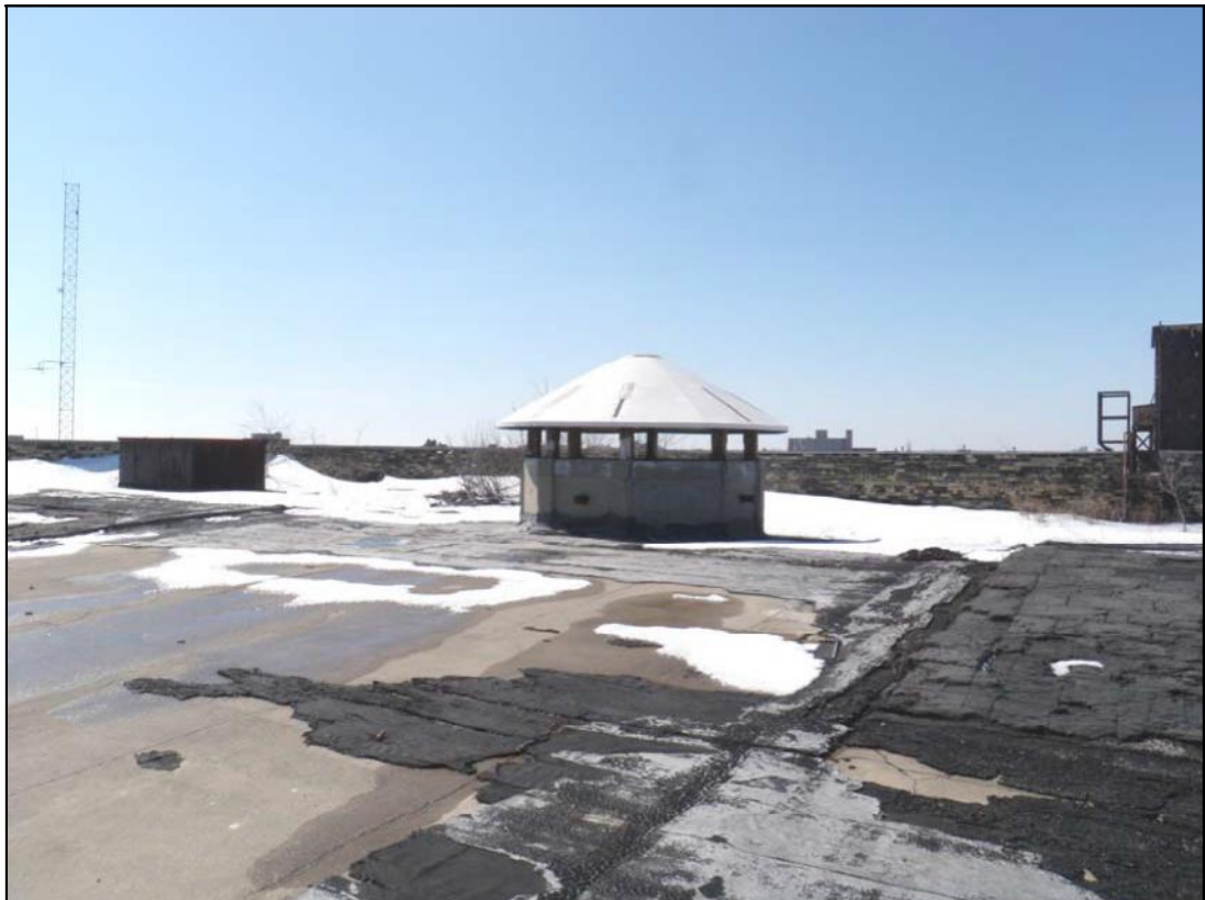
Photo 41: Same looking southwest.
