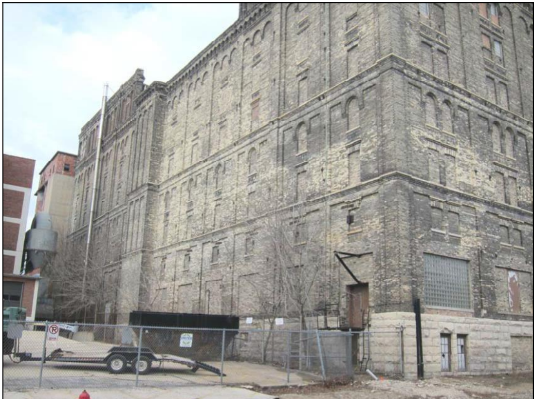
Photo 32: South and east elevations of Building 25 looking northwest.
