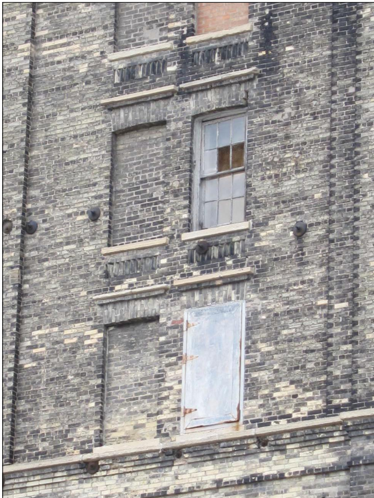
Photo 15: Upper floors of east elevation of Building 25.
