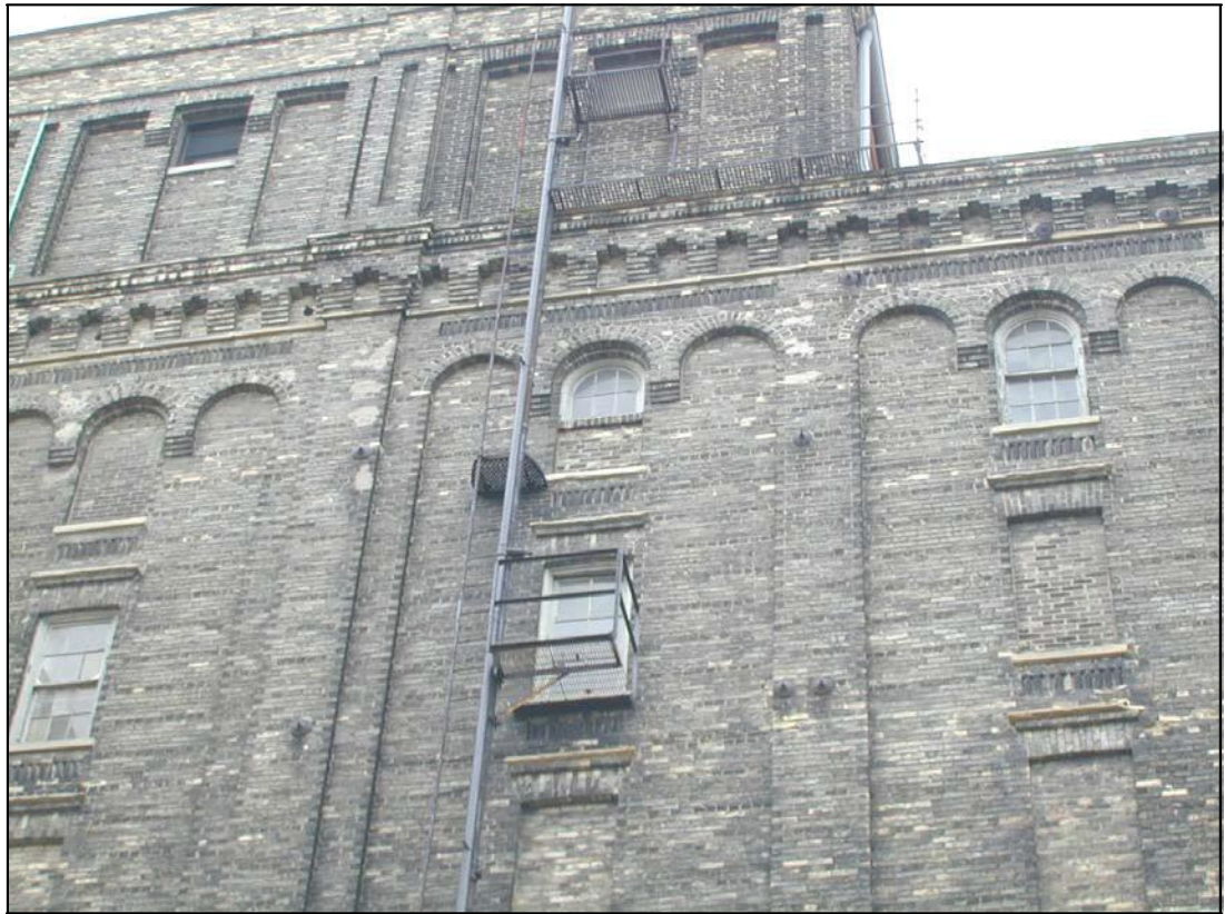
Photo 8: Upper floors of north elevation of Building 25.
