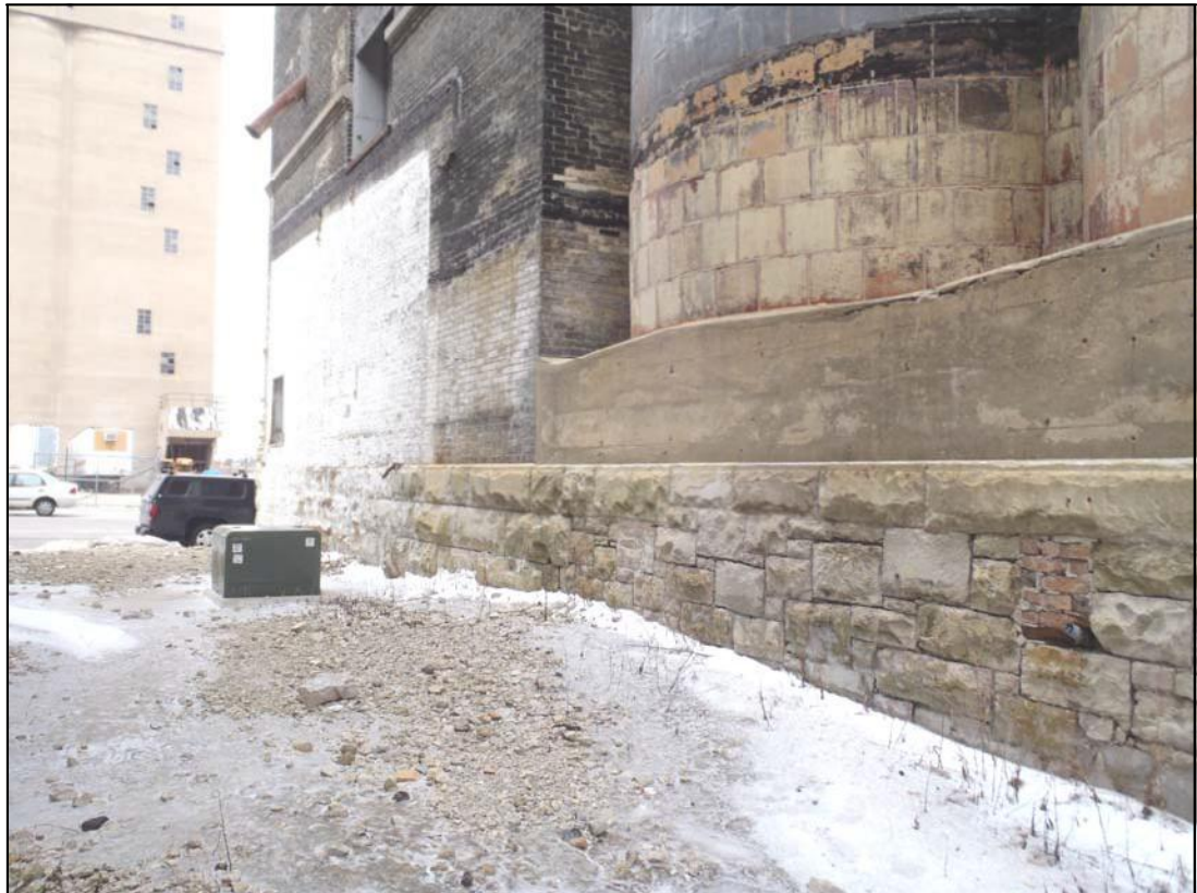
Photo 22: West elevation of Building 24 looking north.
