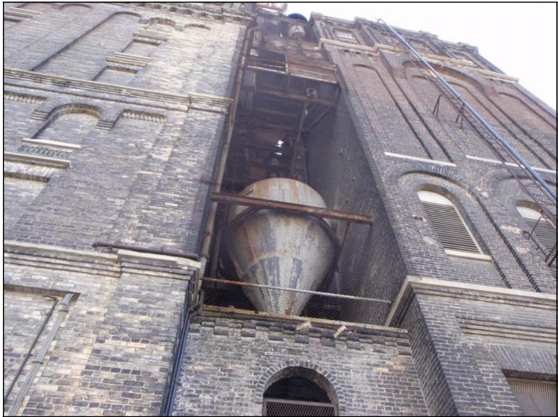
Photo 17: Upper floors of north elevation of Building 24.
