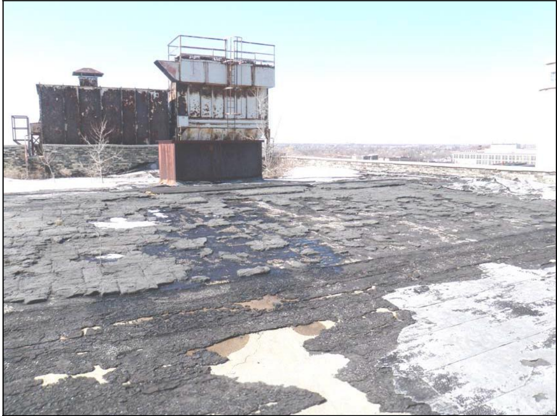
Photo 40: Building 25 roof on seventh floor west penthouse looking northwest.
