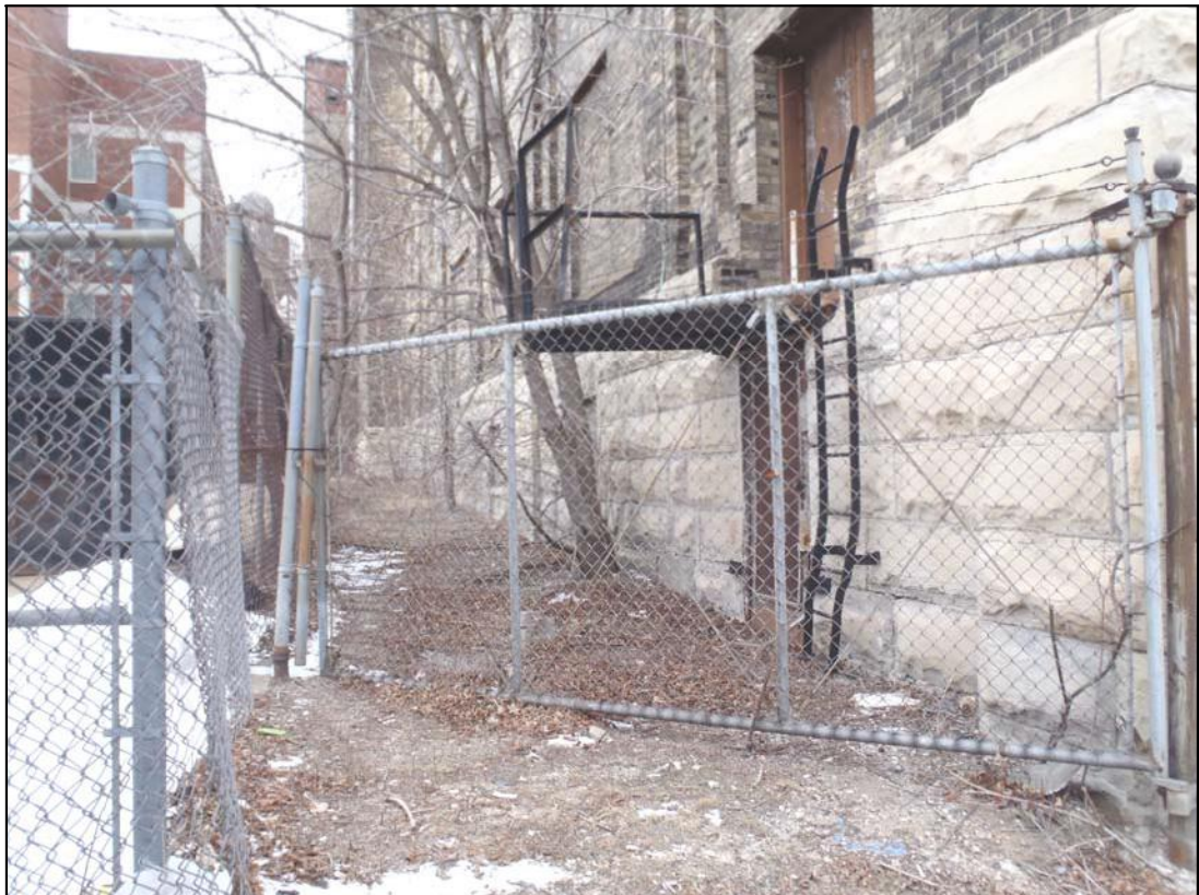
Photo 28: South elevation of Building 25 (right) looking west along property line.
