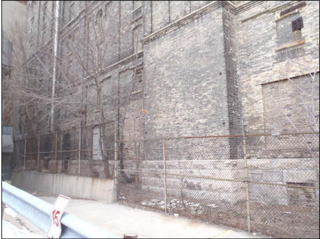
Photo 31: South elevation of Building 25 looking northwest.
