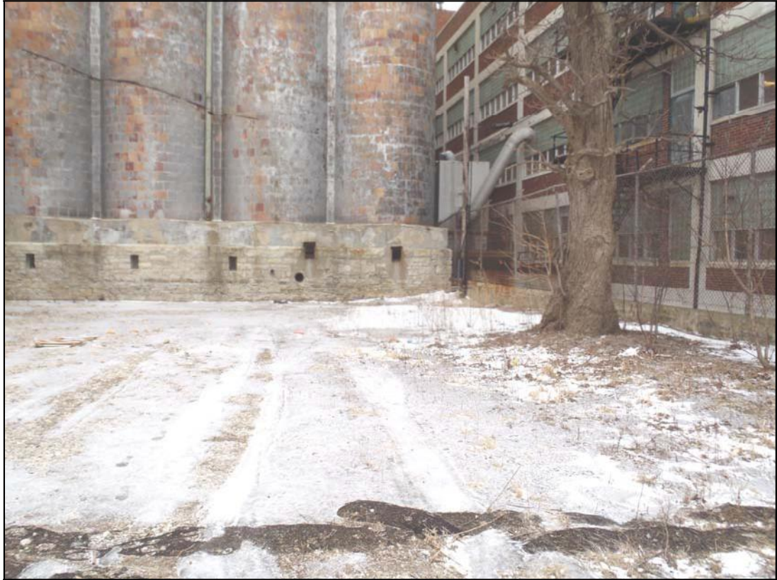
Photo 25: West elevation of Building 24 grain silos looking east.
