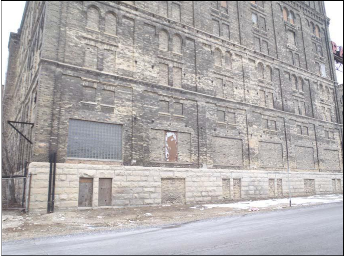
Photo 36: Lower floors of east elevation of Building 25 from across North 10th Street.
