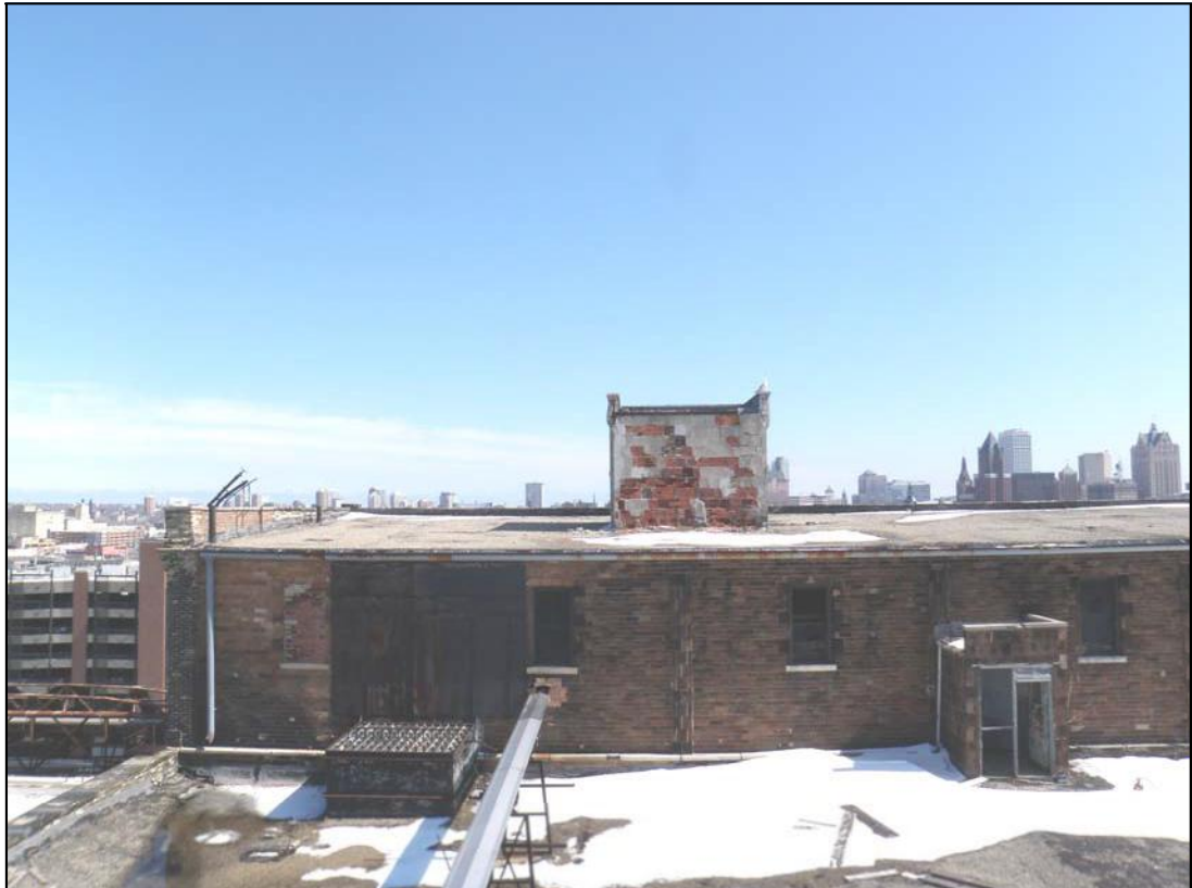
Photo 43: Building 25 roof on seventh floor east penthouse looking east.
