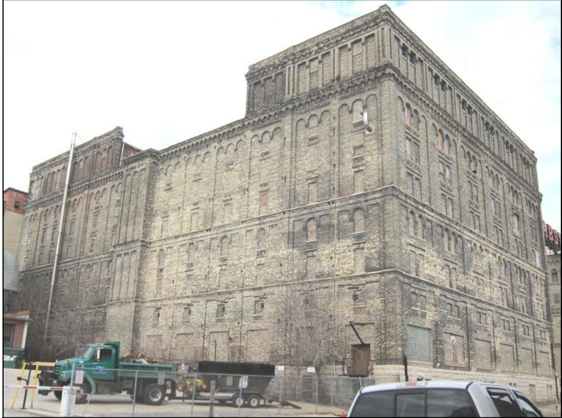
Photo 34: South and east elevations of Building 25 from across North 10th Street.
