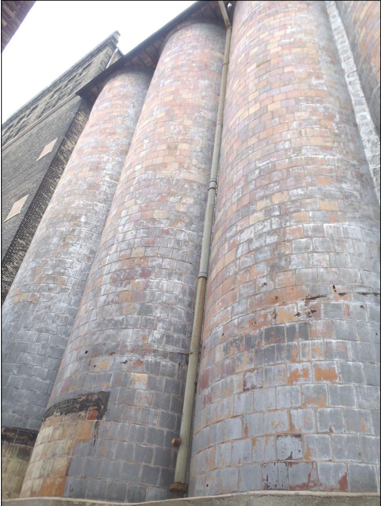
Photo 24: West elevation of Building 24 grain silos.
