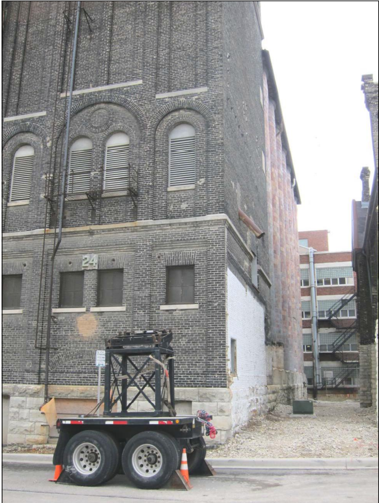
Photo 20: North and west elevations of Building 24.
