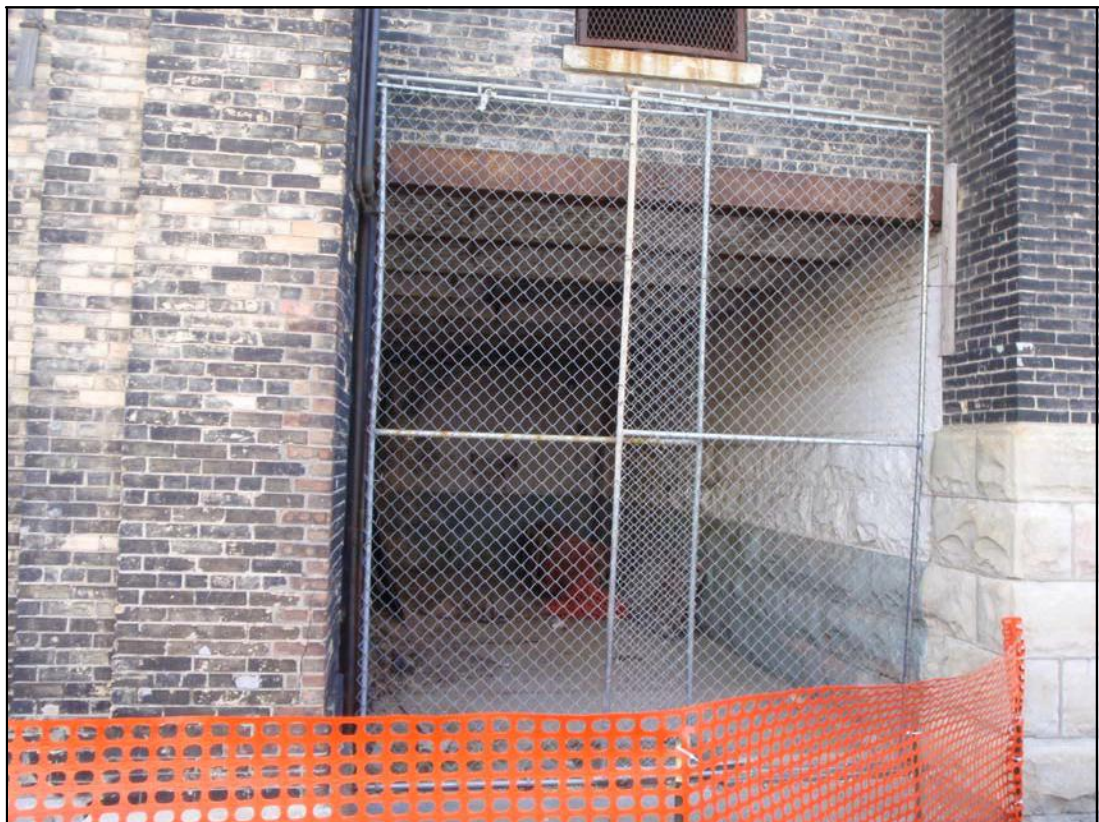
Photo 18: Ground floor of north elevation of Building 24.
