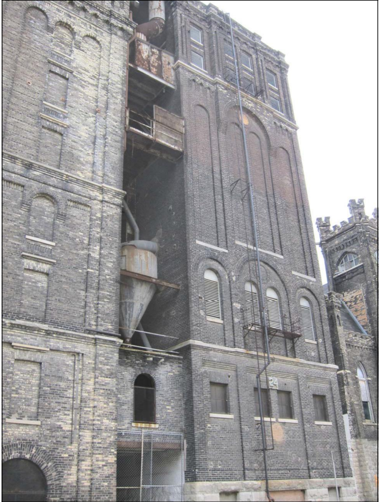
Photo 16: North elevation of Building 24 (center).
