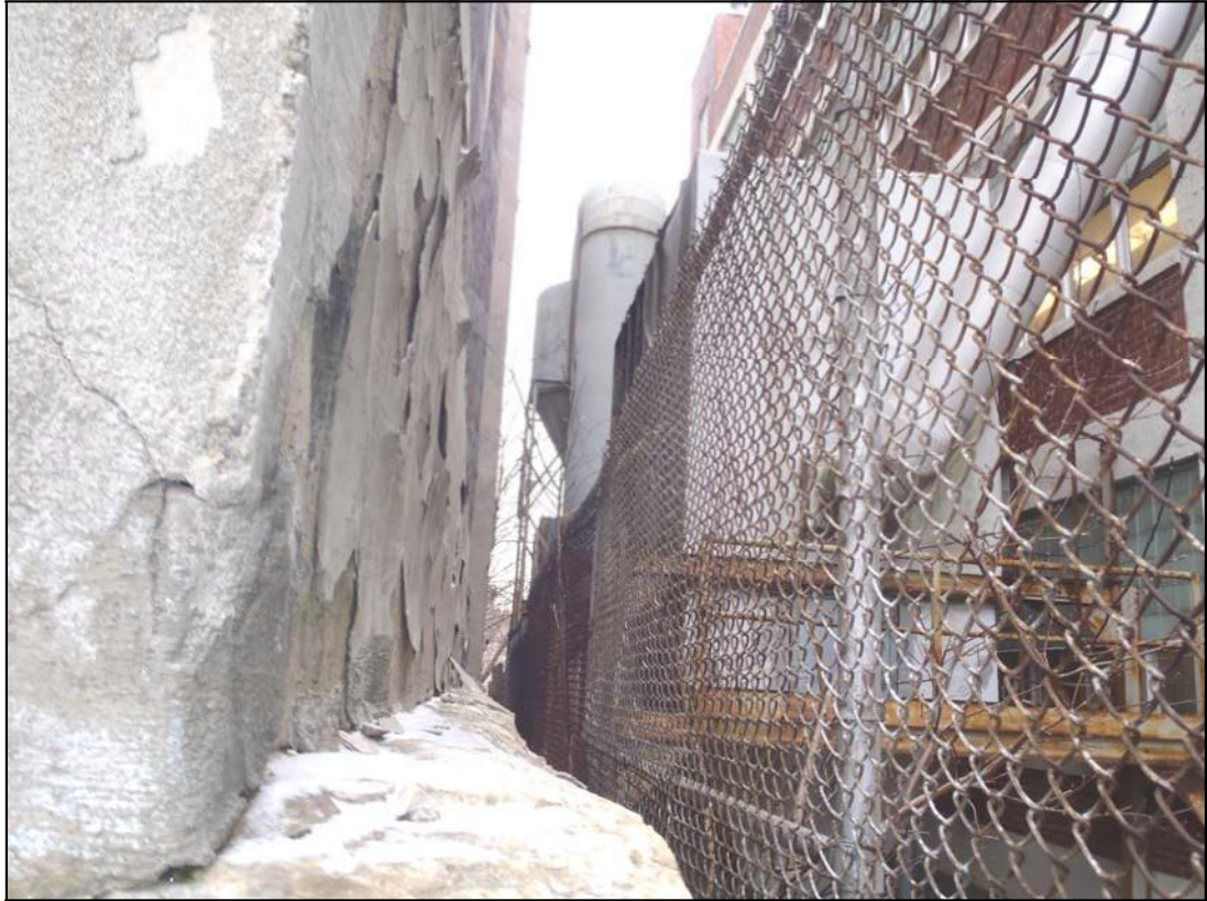
Photo 27: South elevation of Building 24 (left) looking east along property line.
