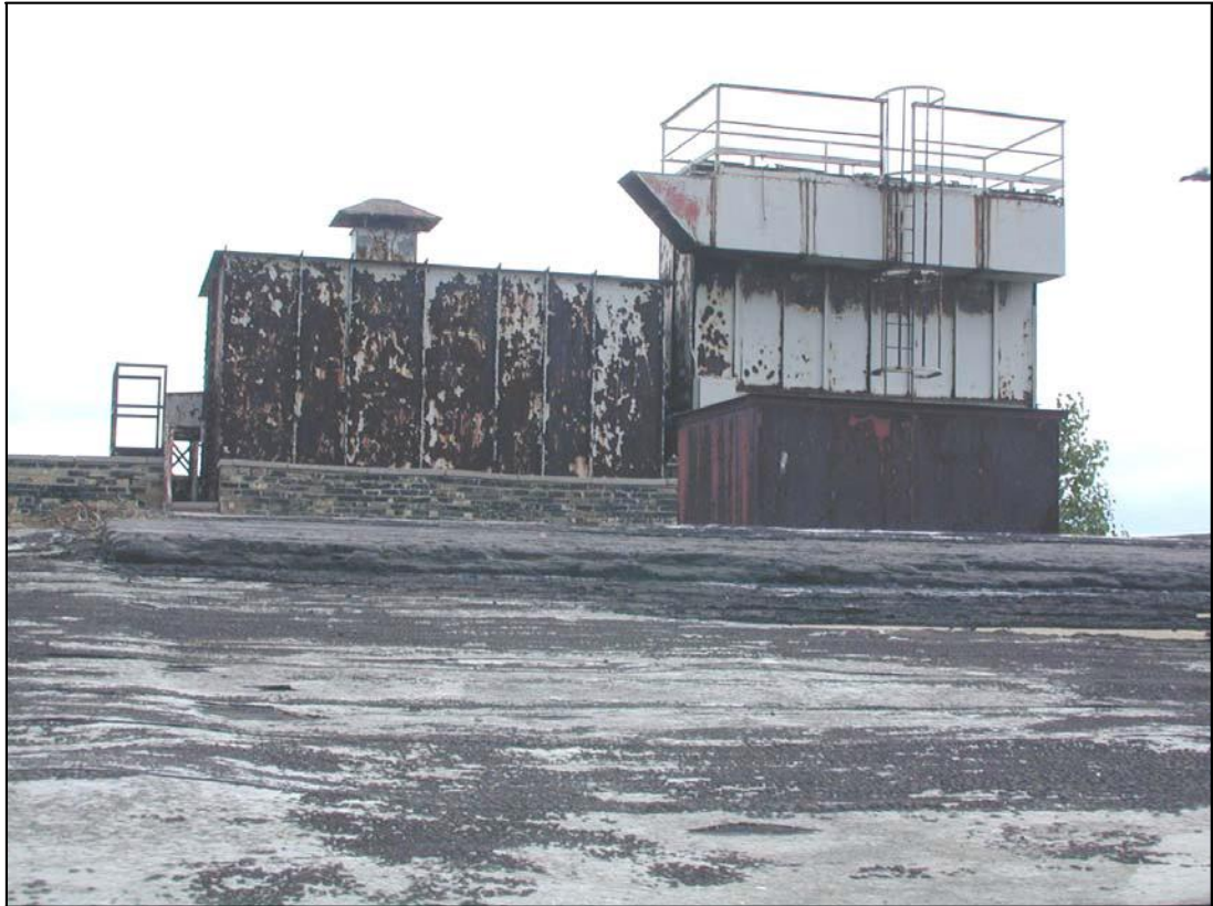
Photo 178: Building 24 roof—looking west from Building 25.
