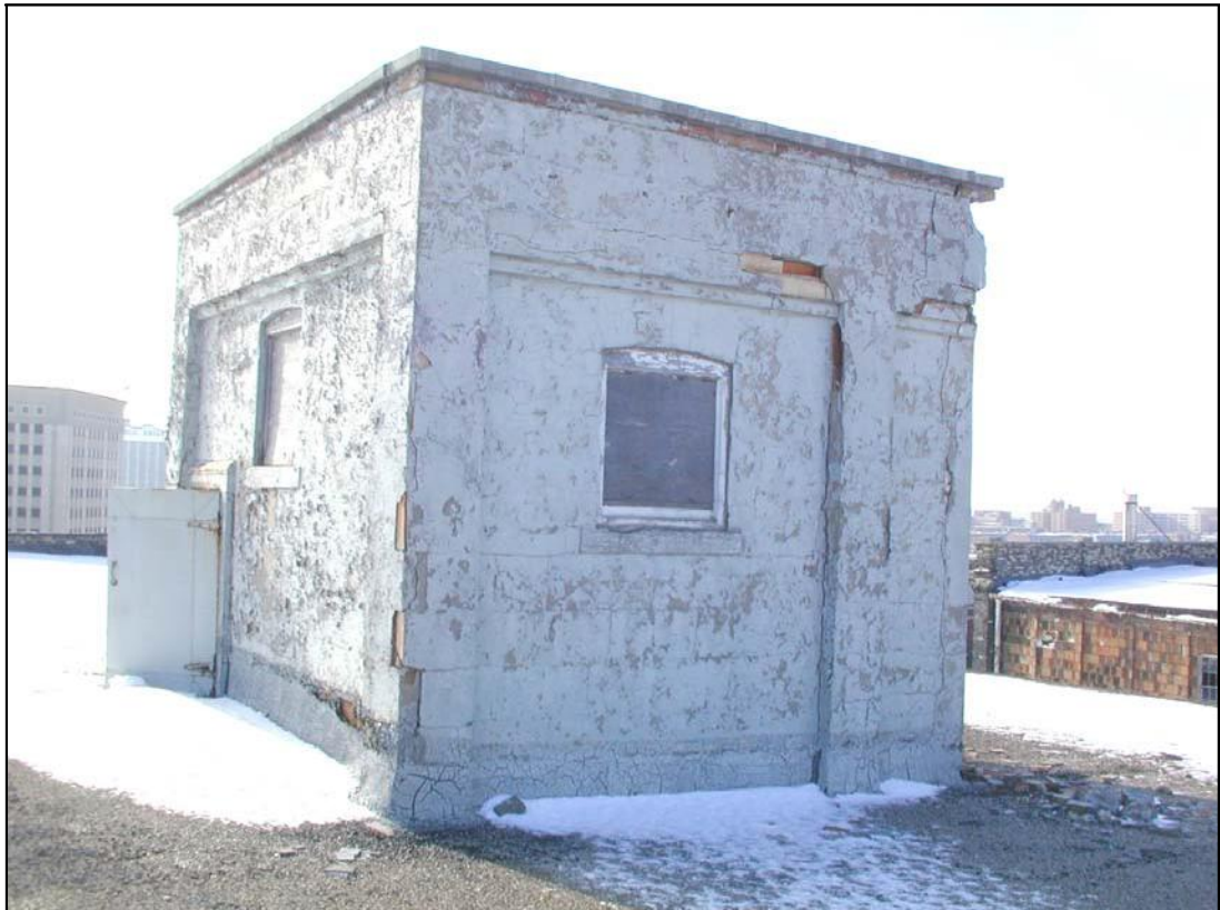
Photo 47B: Same looking southwest.
