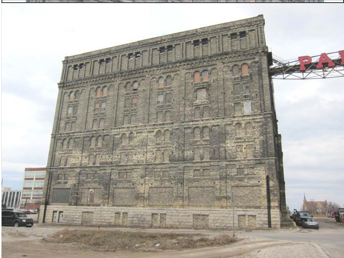
Photo 35: East elevation of Building 25 from across North 10th Street.
