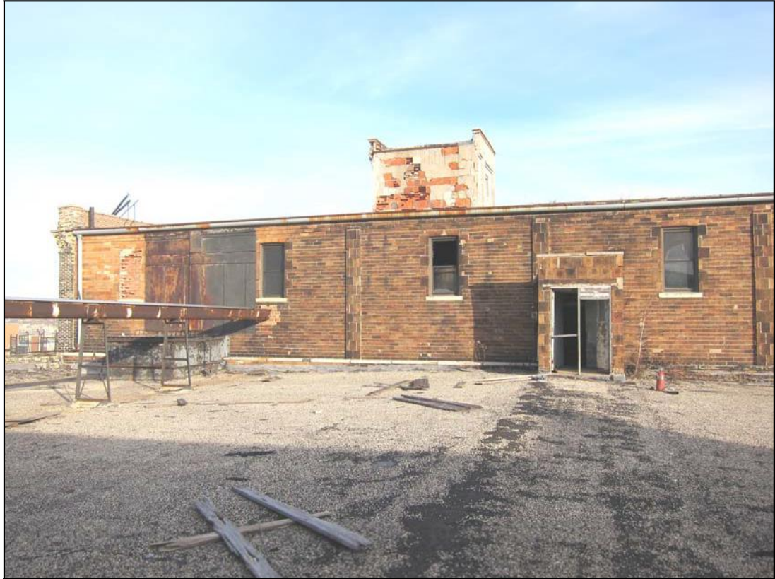
Photo 46: Building 25 seventh floor east penthouse looking east.
