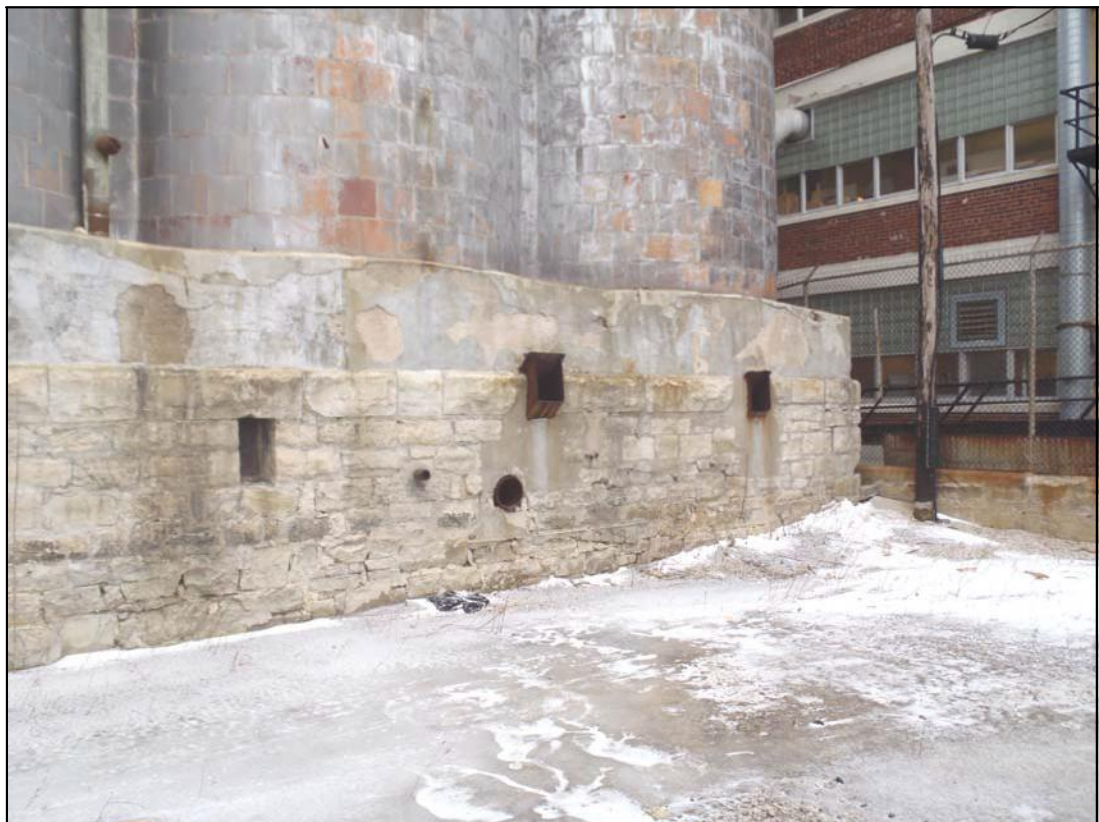
Photo 23: West elevation of Building 24 grain silos looking southeast.
