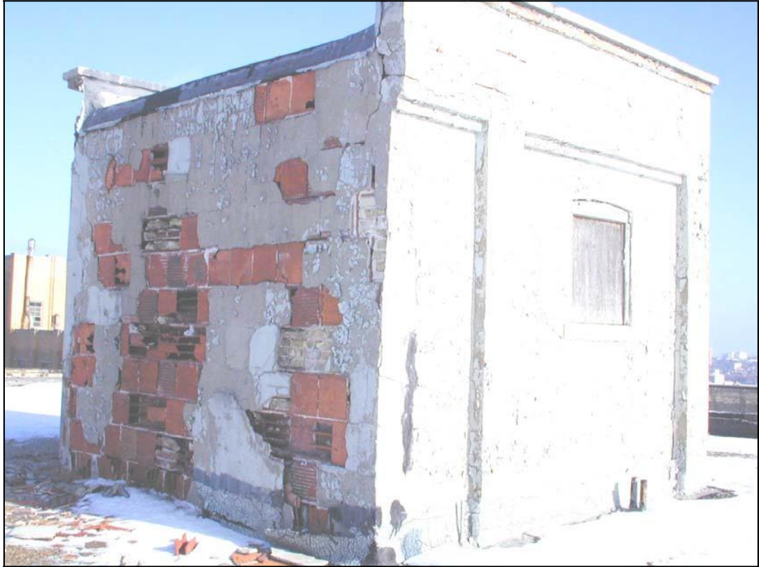
Photo 47A: Building 25 seventh floor east penthouse head house looking northeast.
