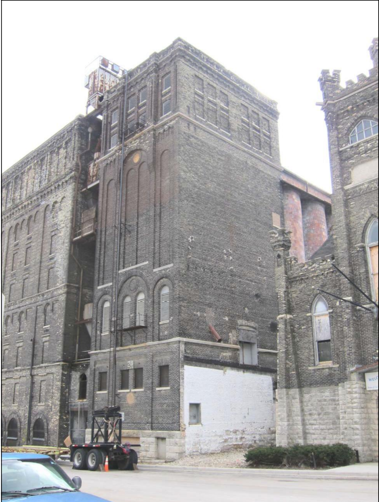
Photo 19: North and west elevation of Building 24 (center).
