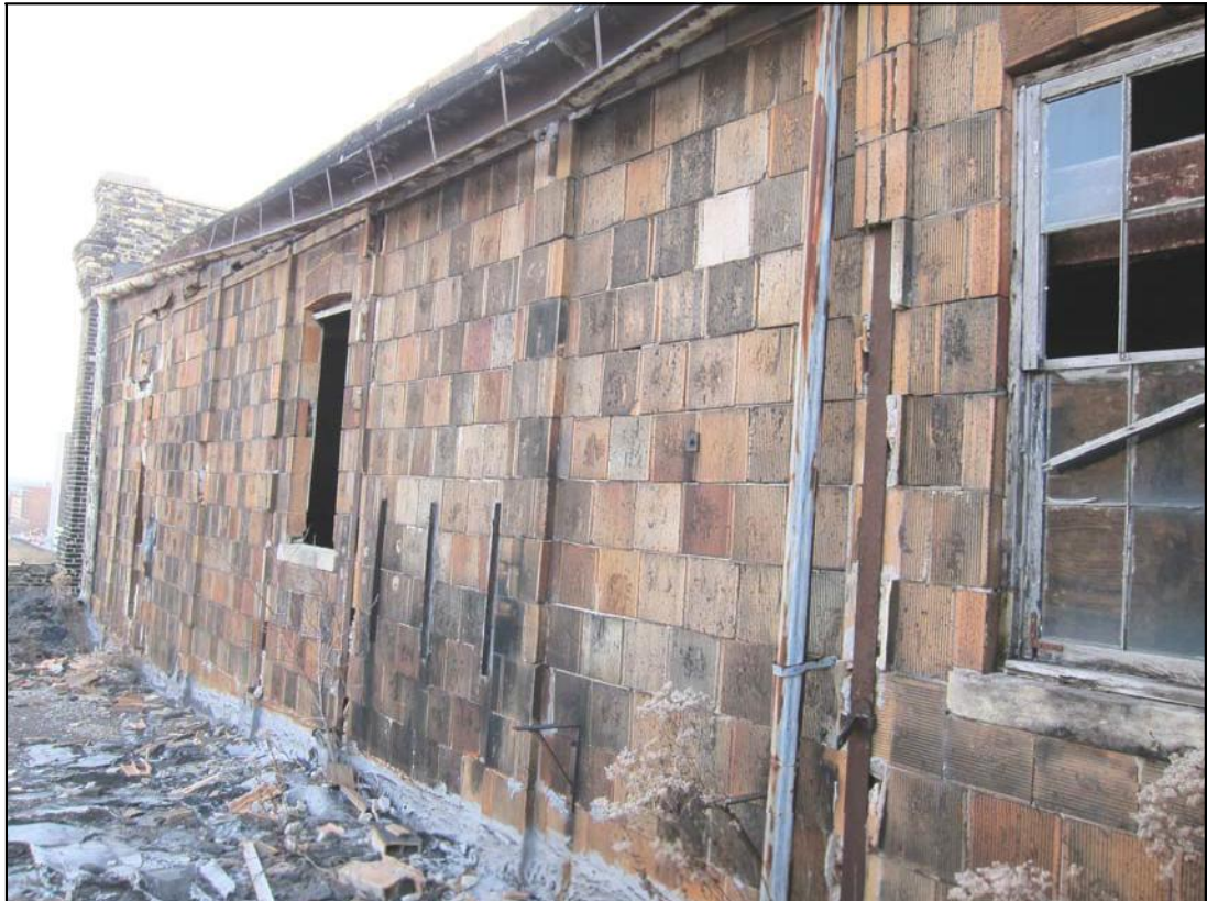
Photo 45: Same looking southwest.
